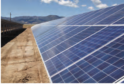
Solar PV panel are fixed angle/position.
