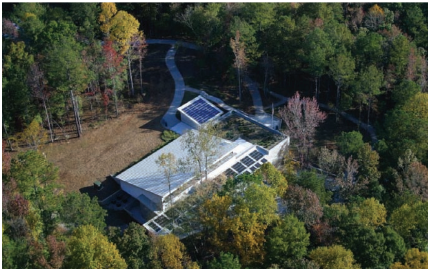
Solar photovoltaic panels on the south-facing portions of the roof generate approximately 20% of the building's electricity.
