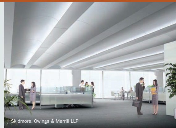
Radiant cooling panels in the ceiling provide cooling; ventilation air is delivered from below the floor.
