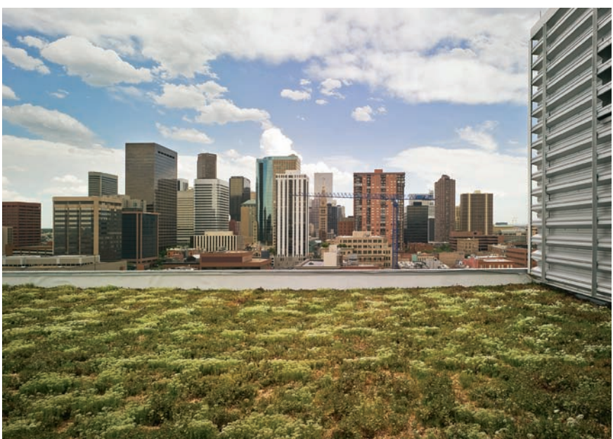
The 20,000 ft 2 vegetated roof (covering three terraced levels) controls storm water, absorbs carbon dioxide and decreases the urban heat island effect. It is the first vegetated roof in Denver used to manage storm water.
