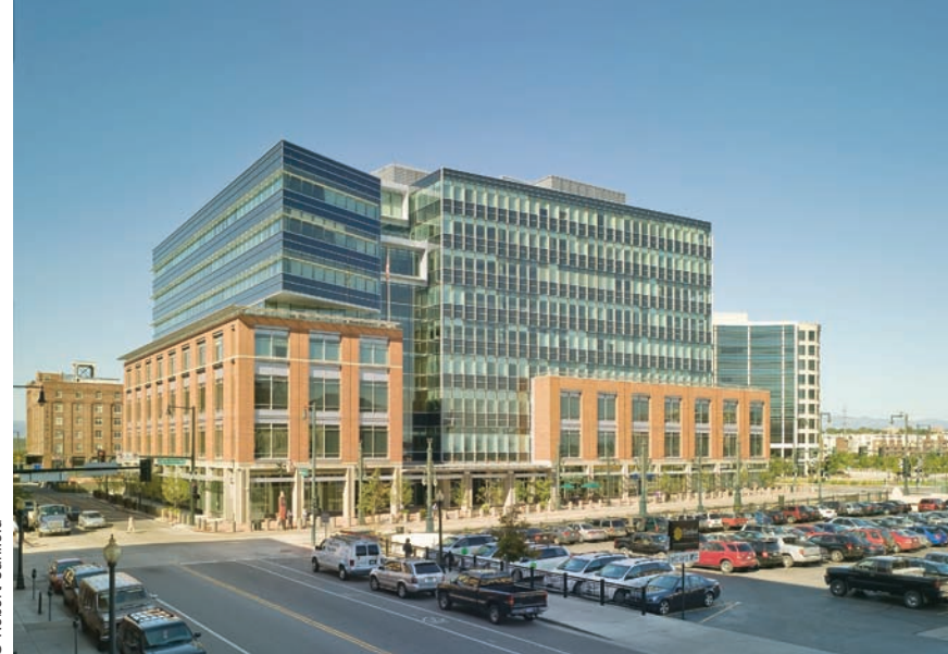
Above The EPA Region 8 Headquarters is a mixed-use building that meets the EPA's security requirements and its mission of sustainability. Energy and daylighting simulation helped the building team design the building's massing and orientation to take maximum advantage of the sunny, dry climate.
