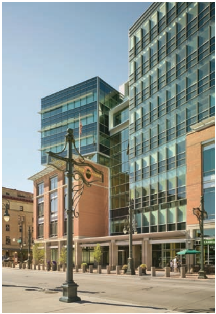
The building's exterior blends the brick façades found throughout Denver's Lower Downtown Historic District with the more modern steel and glass façades of the newer areas of development. Vertical sunshades on the building's northeast and northwest sides block low sun angles during the early morning and late afternoon hours.
