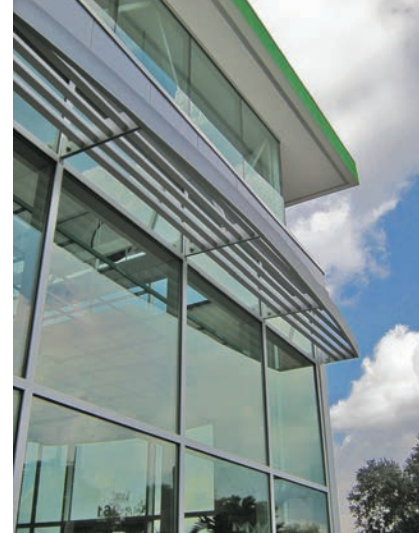
Above The super high-efficiency insulated low-e glass pairs minimal solar heat gain with optimal visible light transmittance. Below The project takes advantage of the existing storm water pond (next to parking lot) and uses the adjacent utility easement on the site by creating a brick-paved plaza that connects it to the outdoor pavilion.
