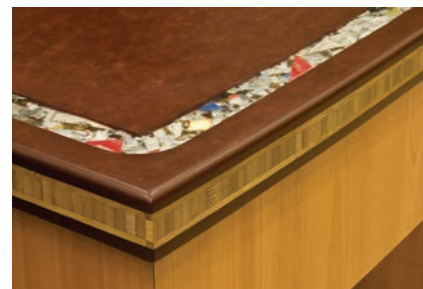
Above Interior finish materials include recycled paper counter tops with inlaid bamboo and recycled credit card details. Left Accessible and flexible "teller transaction pods" eliminate the impersonal physical barriers typically found in other financial institutions.
