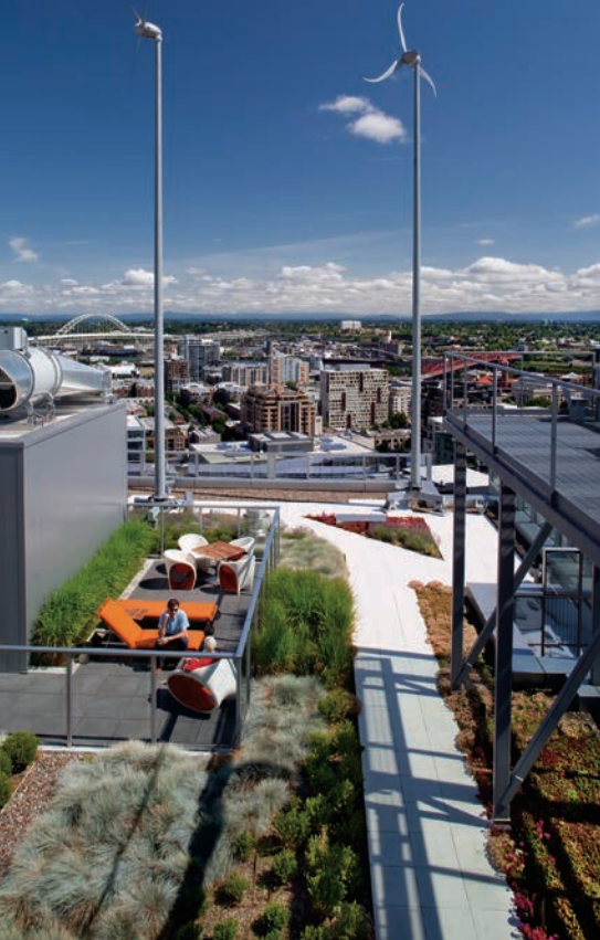
The green roof reduces storm water runoff and the building's contribution to the urban heat island effect, and provides an amenity for the building's residents.
