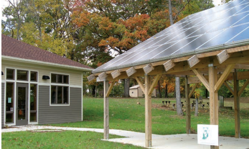
Top The on-site bifacial photovoltaic solar panel installation generates more electric power during a year than the library consumes.
