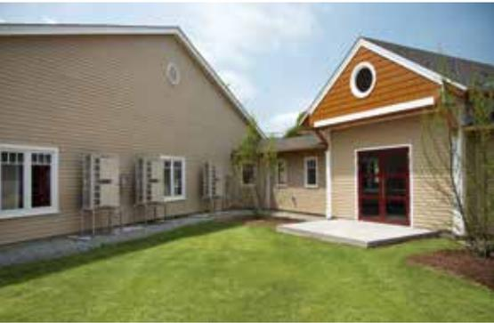
**Clockwise from above** Mechanical equipment is not hidden, rather it is displayed so students can learn how energy is used. The compressors for the air-source heat pumps are on racks to keep them above the snow. Mechanical rooms are not necessary for this type of equipment.
