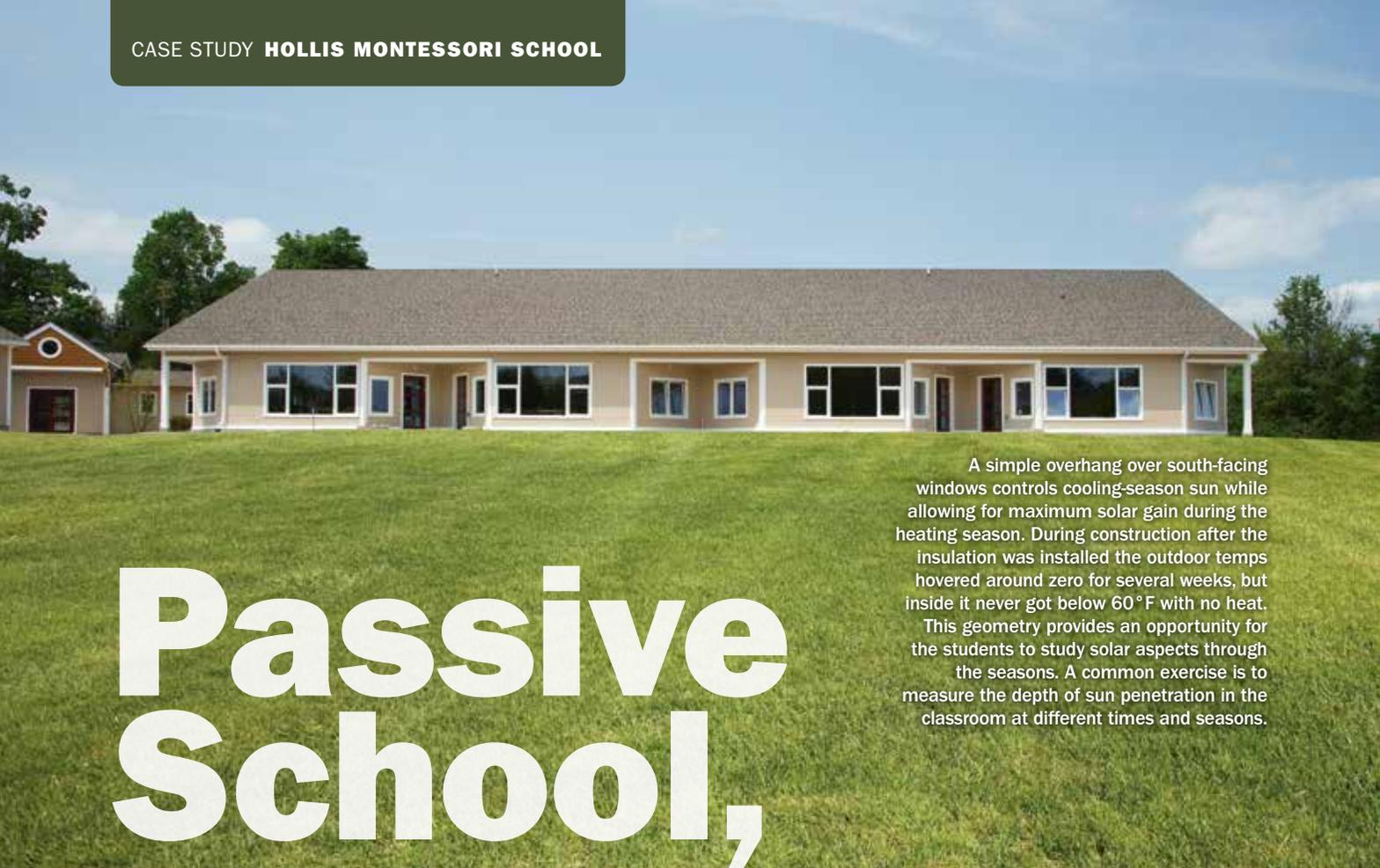
A simple overhang over south-facing windows controls cooling-season sun while allowing for maximum solar gain during the heating season. During construction after the insulation was installed the outdoor temps hovered around zero for several weeks, but inside it never got below 60°F with no heat.
