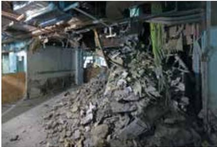
**Clockwise from above** The gut renovation of Sherman Fairchild was achieved through extensive demolition. Over 90% of waste materials were diverted from a landfill.
